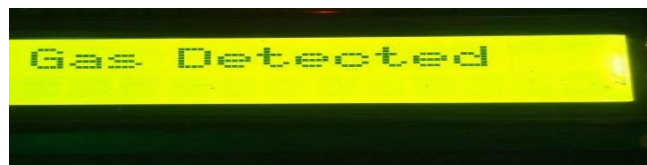
Fig. 12. LCD display showing hazardous gas detection alert
